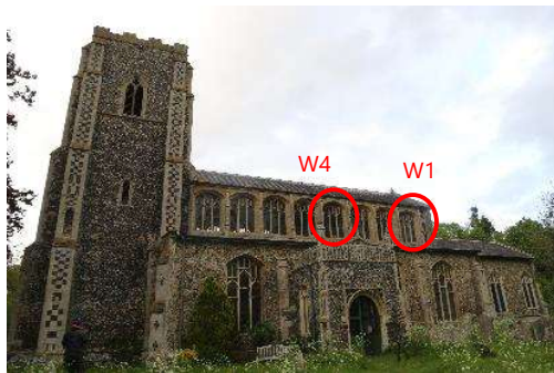
Figure 1. South aisle exterior. Overstorey windows with missing pane of glass used as a primary bat access into church interior.
