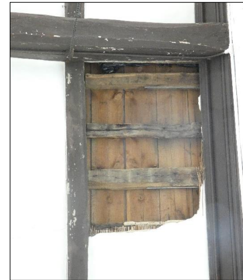
Photograph 9.2.6: The hole in the ceiling of the nave.
