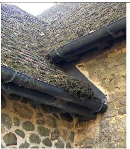
A very blocked gutter may lead to damp problems. Check the corresponding area inside the church to make sure this has not occurred
