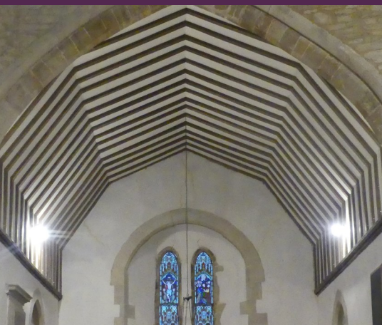
False chancel ceiling with bat void St Lawrence, Radstone
