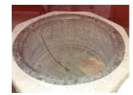
Lead is most likely to be found on monuments as an infill to lettering or as a liner to fonts. Lead is also historically used to fix ironwork to masonry and so may be found around the ends of railings.
