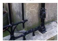
Iron is most commonly used for railings, window ferramenta, or structural restraints. It is often painted although it may be in a rusty condition especially where it meets stonework. If unsure, iron and steel are both ferrous and can be identified with a magnet.
