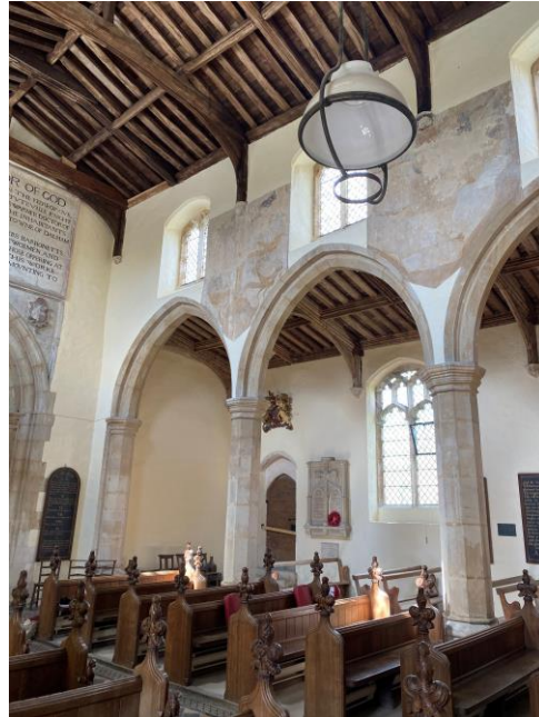
Photograph 4 Chancel and north aisle
