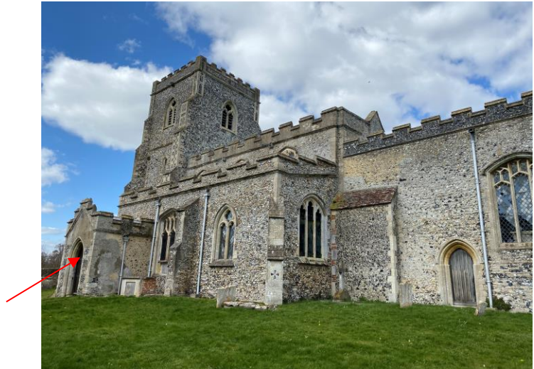
Photograph 1 Southern elevation of church, with main access location for bats at the porch shown by the arrow
