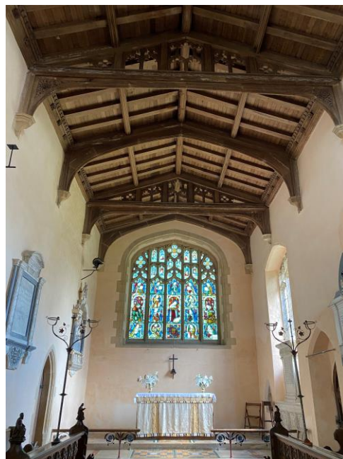
Photograph 3 Interior of church chancel
