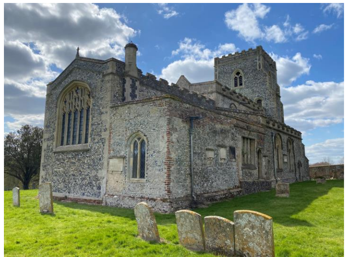
Photograph 2 Eastern and northern elevations of church
