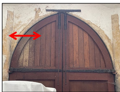
Figure 12 – Main access into the church via the western tower door. The bats have worn the staining off the door. Copious amounts of droppings are present at the base of the door
