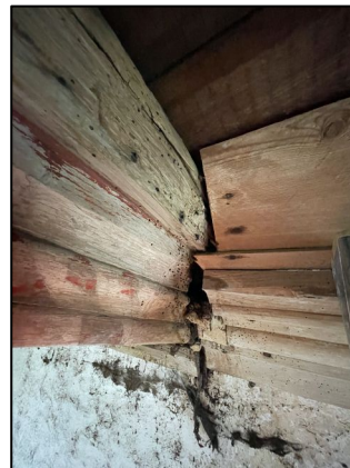
Figure 24 – Gap beside principal rafter in the south aisle to be repaired. There was no evidence of bat roosting in this area and the works to this should remove future potential
