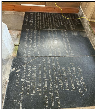
Figure 21 – Ledger stones in the south aisle – evidence of current and historic urine damage
