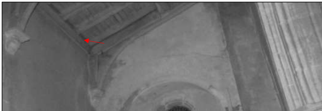
Photograph 3.1.10: The Natterer’s bats (re)enter the church via gaps at the wall plate of the north aisle. The red arrow shows an internal view of one of the three features used (feature 4b, Figure 10.1), in the north-east corner.
