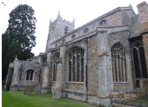
Figure 3. Southern aspect of the church, showing the south aisle, southern porch and the tower.
