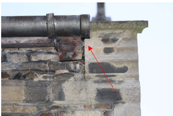
Bat access points via eaves on south side of chancel
