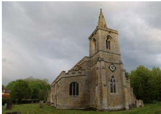
Figure 1. Western elevation of the church, showing clocktower and spire, and the north aisle, with the nave centrally.
