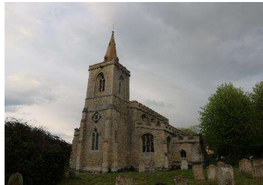
Figure 2. Western elevation of the church showing the tower and spire, and the south aisle and porch, with the nave centrally.
