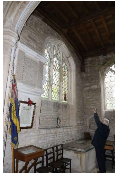
Figure 9. The western end of the north aisle.
