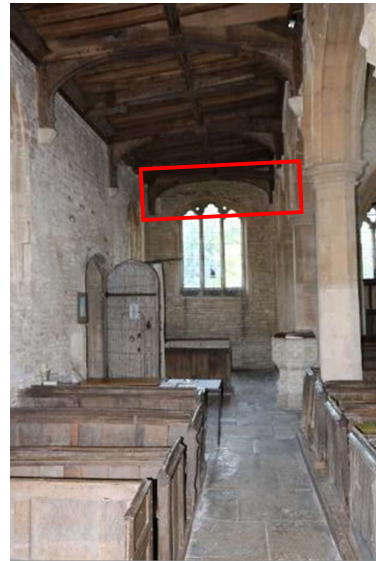
Figure 6. Internal view of the south aisle, looking westwards with the kitchenette in the background. The secondary pipistrelle roosting location is highlighted (red).
