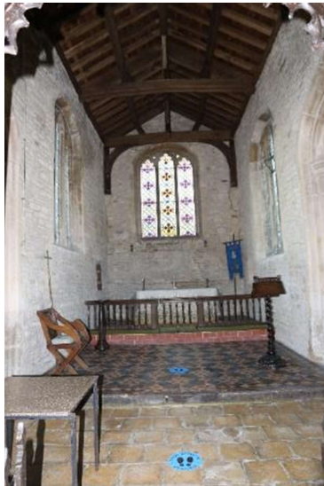
Figure 5. Internal view of the chancel, showing timber structure.
