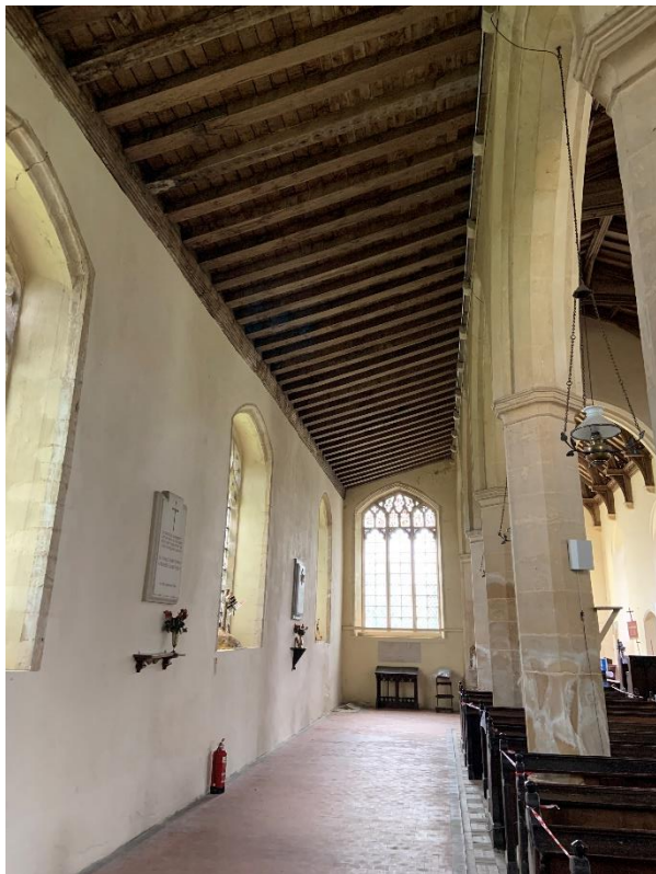
Photo 6. North aisle (from west end facing east).
