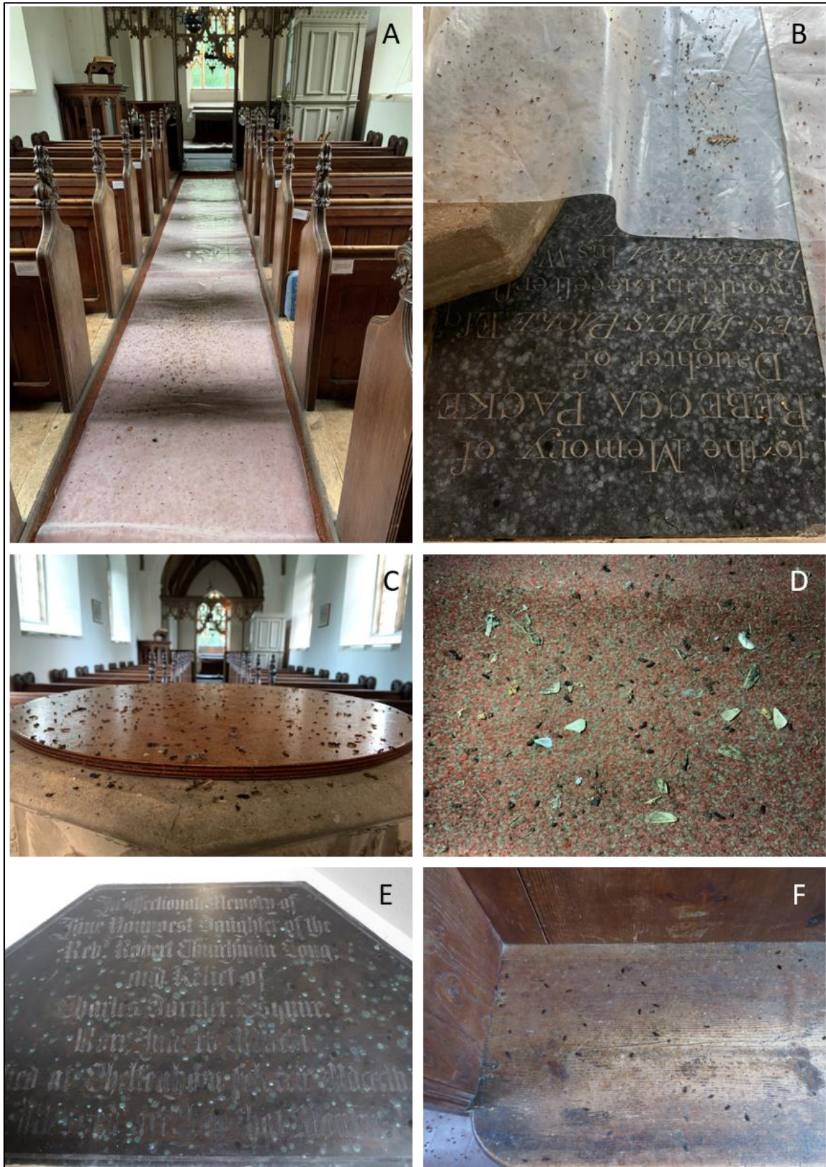
Figure 5. Photos illustrating some of the impacts of bats on the church. A. Plastic sheeting on the nave floor, with bat droppings and urine. B. Bleaching to ledger stone from bat urine. C. Bat droppings on the font. D. Brown long-eared bat feeding remains (moth wings) and droppings. E. Bat urine bleaching on a wall memorial. F. Bat droppings and urine bleaching on a pew.
