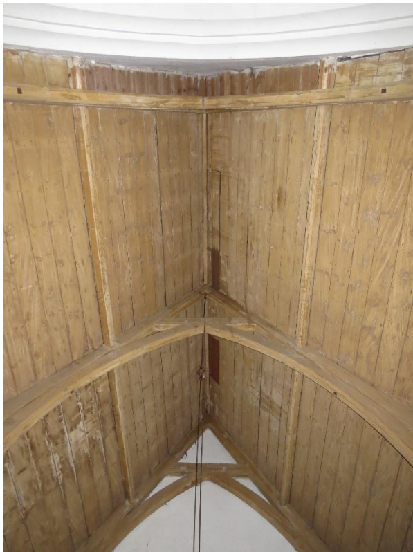
Photo 6. Chancel roof interior.
