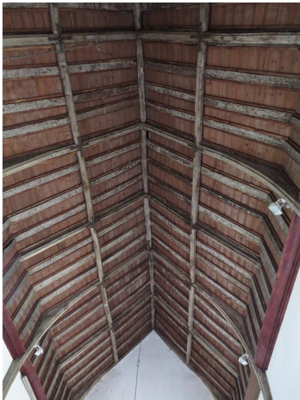
Photo 4. Nave roof interior.
