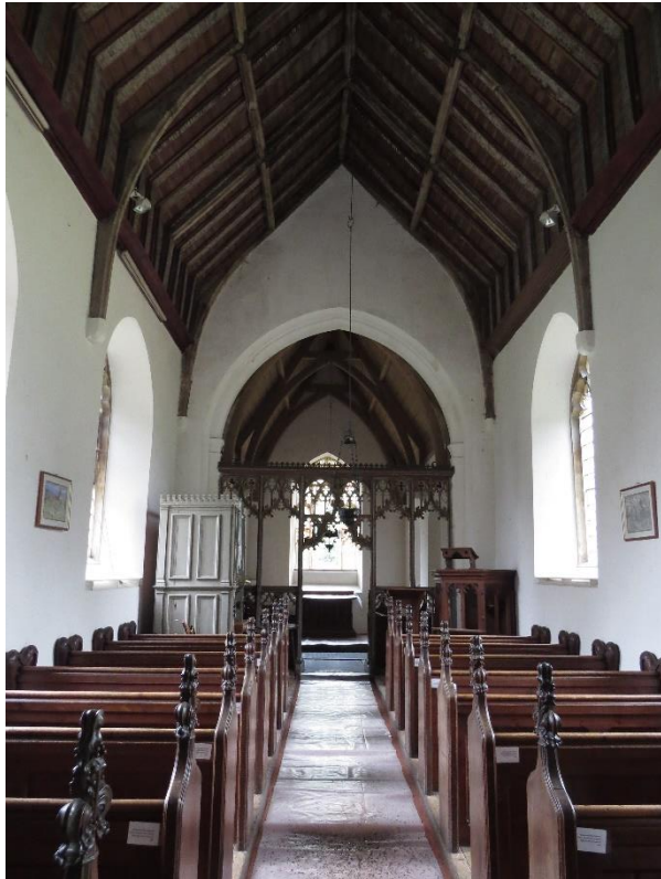
Photo 3. Nave interior (from west end facing east).
