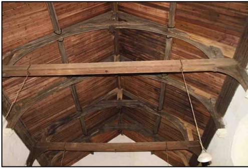
Figure 14 – General view of the nave roof
