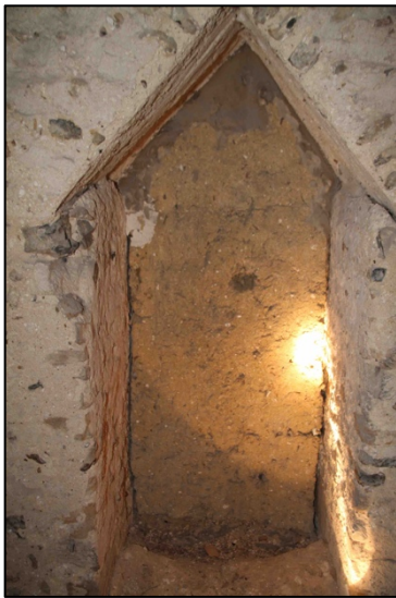
Figure 22 – Sealed window into the nave
