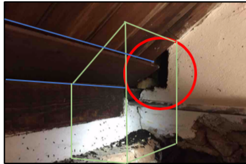
Figure 19 – Bat access and bat box in the south-west corner of the nave – the common pipistrelles access the church in this location. The soprano pipistrelles use the box for roosting but also access between the boarding and the roofing felt as far as the principal rafter. Occasional soprano pipistrelles access the main body of the church for flying. It would be useful to be able to make the board (highlighted blue) removable to clear out droppings from the roosting area. A possible extension to the box is shown in green
