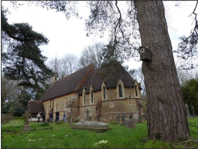
South side and east end showing difference in height between nave and chancel.
