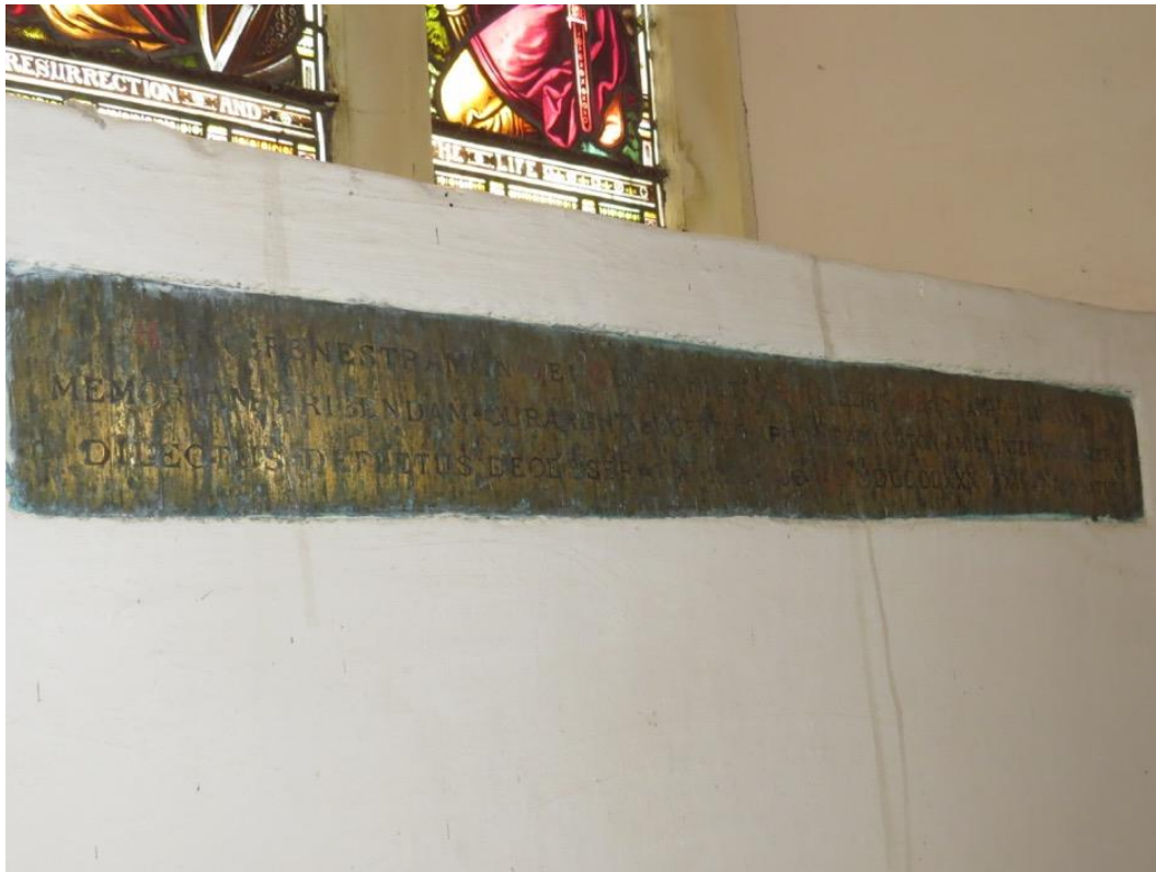
Photo 11. Bat urine staining to brass wall plaque.
