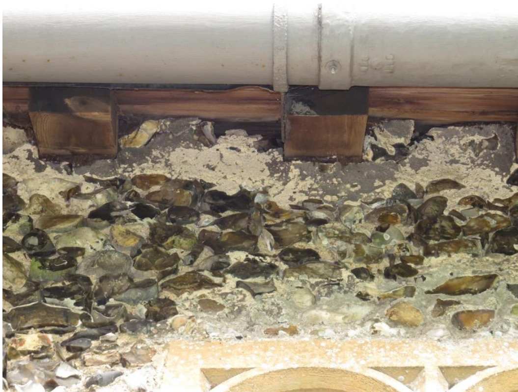
Photo 4. Typical eaves-level bat access point via missing flints/mortar around protruding rafters.
