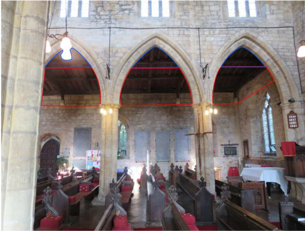
Photograph 27. The north aisle (view to north) showing the edges of the temporary ceiling (red) and the extent of the raised edges (blue)
