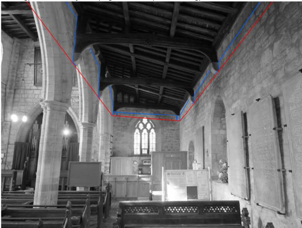
Photograph 26. The north aisle (view to west showing the edges of the temporary ceiling (red) and the extent of the raised edges (blue)
