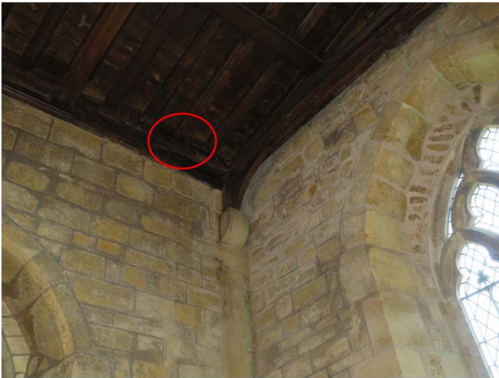
Photograph 19. Daubenton's bat roost above the timber sarking at the north-east corner of the north aisle
