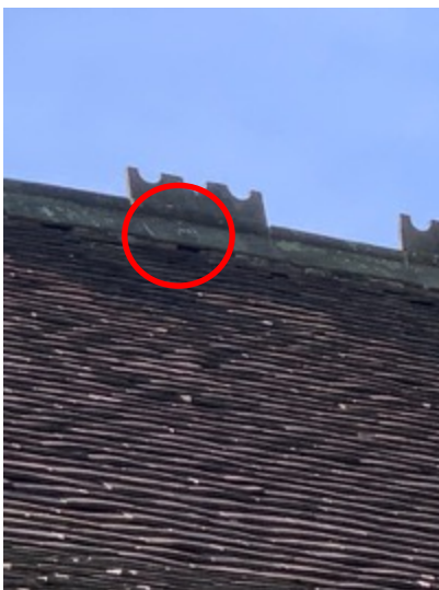
6. North aspect: possible access to interior under roof ridge down length of roof
