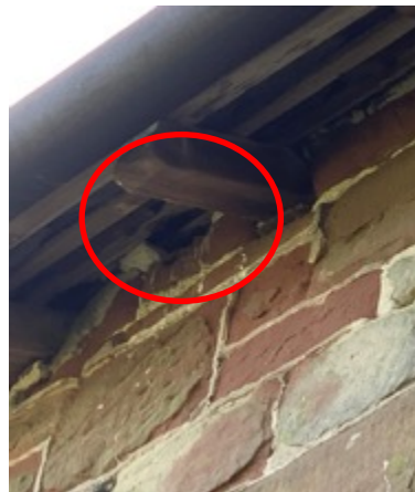
6. North aspect: possible access to interior under roof ridge down length of roof
