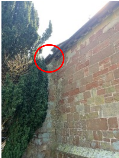
5. Northern side: mortar fallen away under guttering
