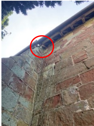
5. Northern side: mortar fallen away under guttering
