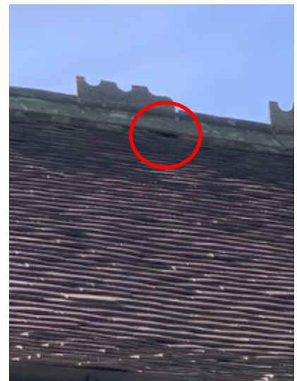
6. North aspect: possible access to interior under roof ridge down length of roof
