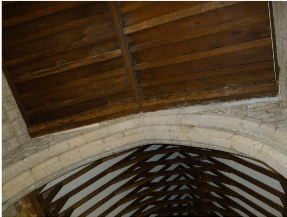
Photo 17 Nave and chancel roofs
