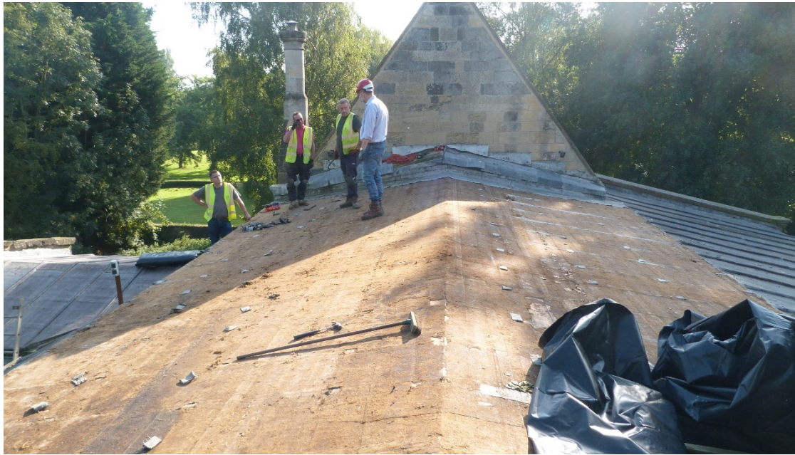
Photo 1 Temporary roof cover being fitted over nave May 2020
