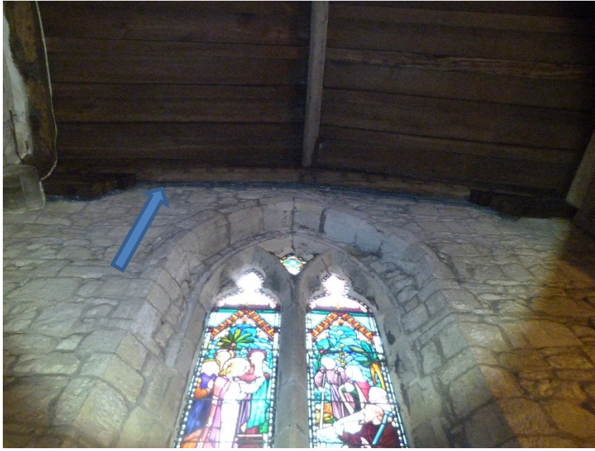
Photo 2 Location of wire mesh west end of nave
