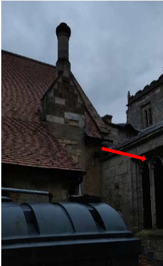
Figure 7 Mnat emergence location north of vestry
