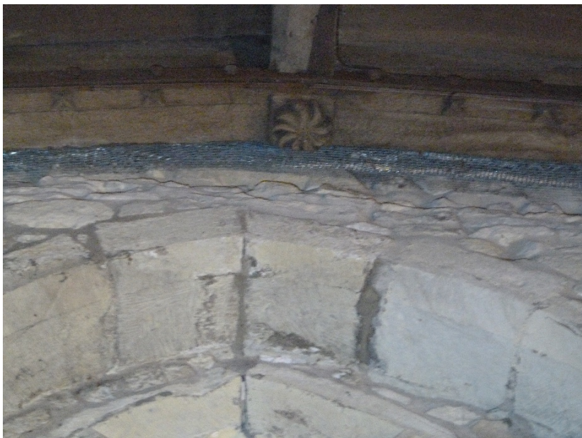
Photo 3 Detail of wire mesh at west end of nave
