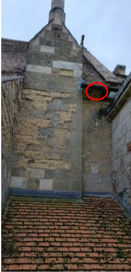
Photo 15 Close up view of vestry access location
