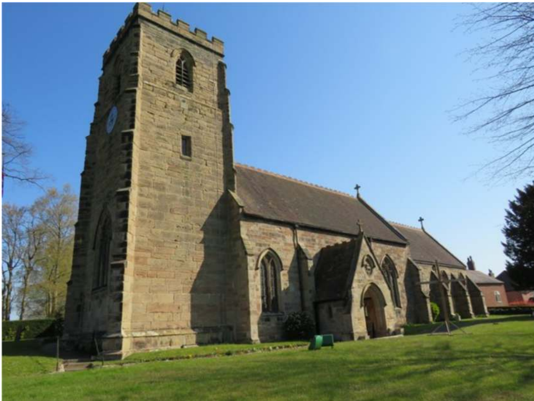
Photograph 1. Church of St Peter, Netherseal (south elevation).
