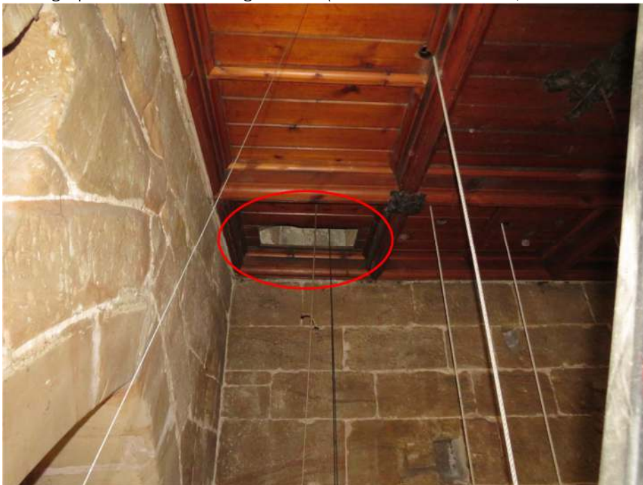
Photograph 23. The clock weight hatch (from the base of the tower)
