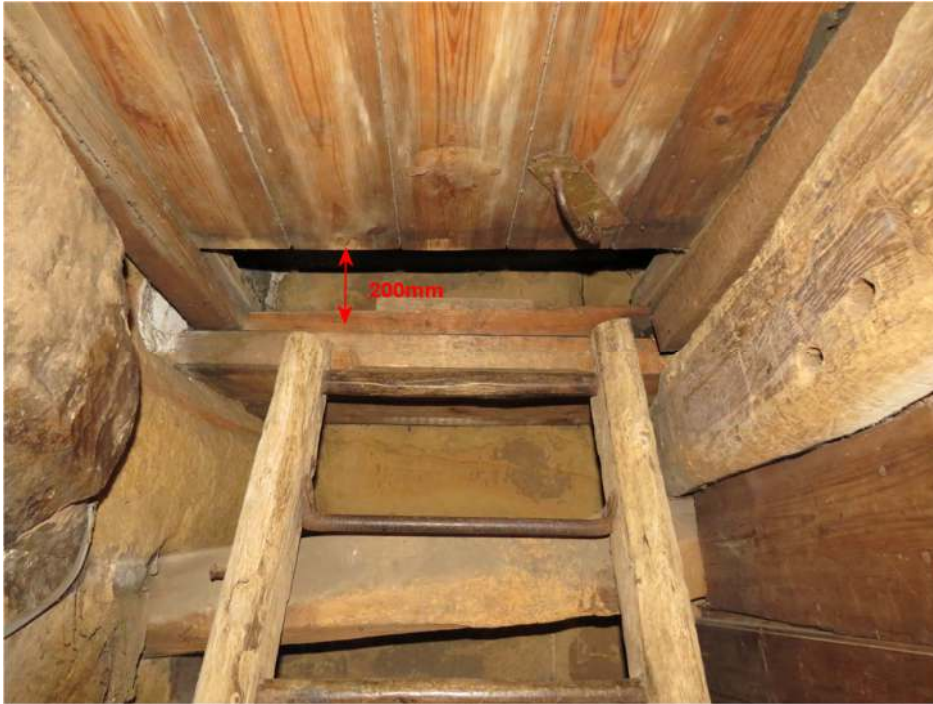
Photograph 24. The access hatch to the belfry showing 200mm gap
