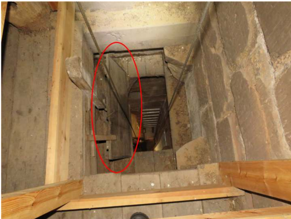
Photograph 22. The clock weight hatch (from inside the silence/clock chamber)
