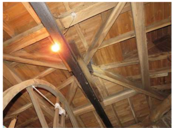
Photograph 9. The underside of the roof within the belfry
