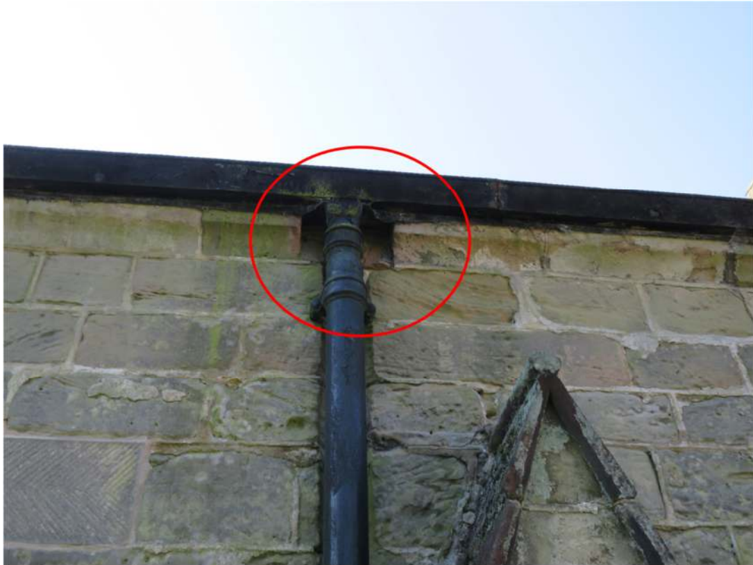
Photograph 20. Access point at top of drainpipe (see Photograph 18)
