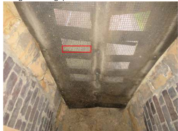
Photograph 24. The access hatch to the belfry showing 200mm gap
