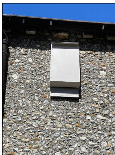
Figure 7 – Triple slot Kent Box installed on a south nave wall
