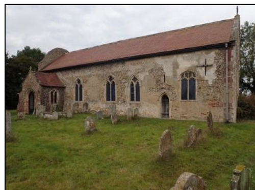
Figure 14 – View of the nave roof and the top of the rood screen. The common pipistrelle's roost in various locations within the nave roof structure
