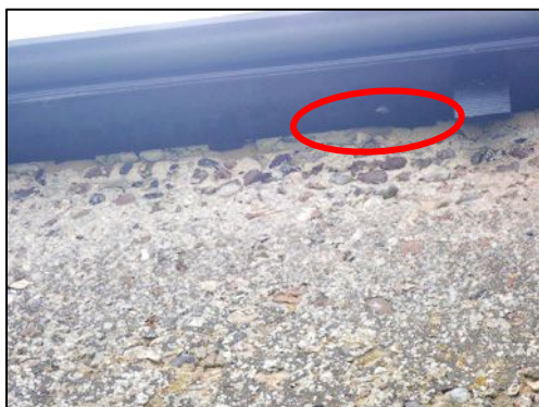
Figure 13 – Location of bat boxes and principal access A1 (red) in the north-west corner of the church
