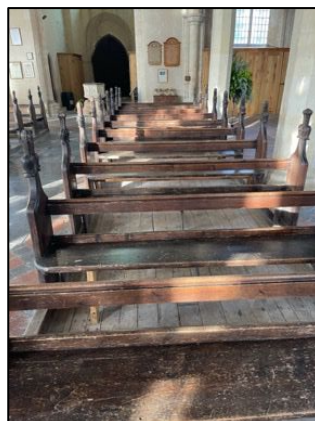
Figure 22 – Medieval pews in the nave. These show significant urine staining
