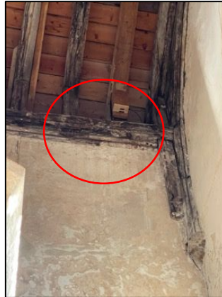
Figure 3 – Internal mortise box installed in the nave. Others were installed in the tower
