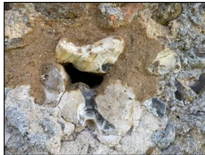
Figure 6 – One of the newly installed putlog holes
