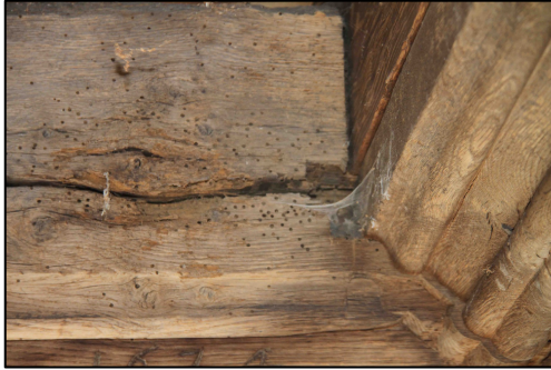
Figure 18 – Timber gap in parvise re-leaded in 2015, no bat evidence in parvise
