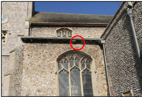
Figure 8 – Secondary access area in the south-west corner of the south aisle
