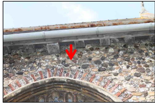
Figure 7 – Secondary access eaves detail on the south aisle showing the overhang and exposed rafters from which a small number of bats emerge
