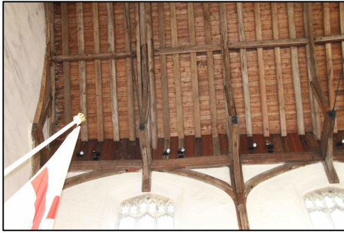
Figure 24 – Roof structure close to principal access
