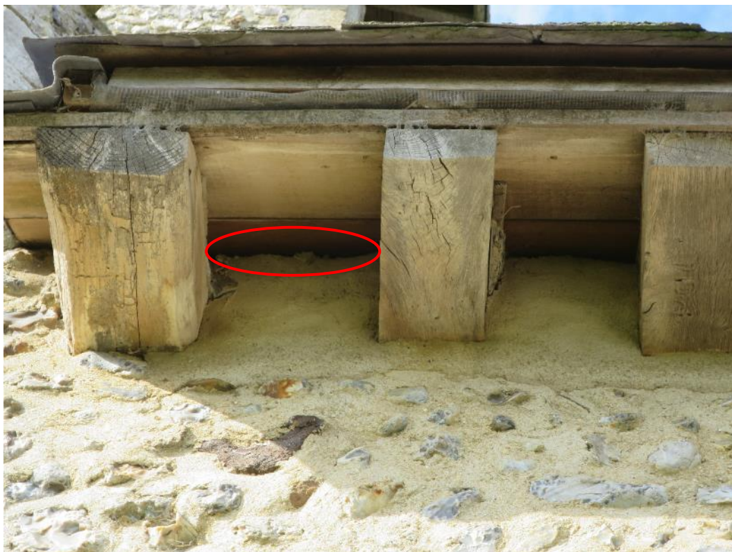
Photo 10. Typical access to/from the outside at eaves (circled in red).
