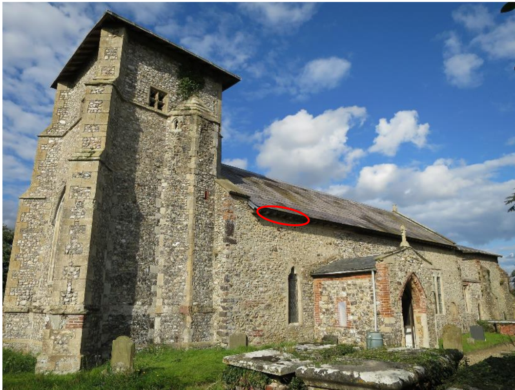
Photo 1. Southern elevation (main access circled in red).
