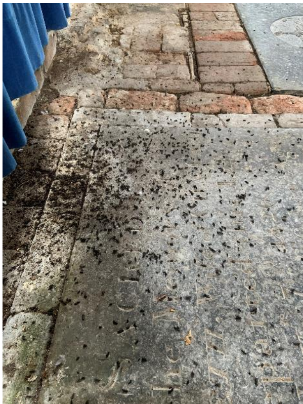
Photo 12. Bat droppings at west end of nave (beneath roost B, Figure 7) with staining/bleaching to ledger.
