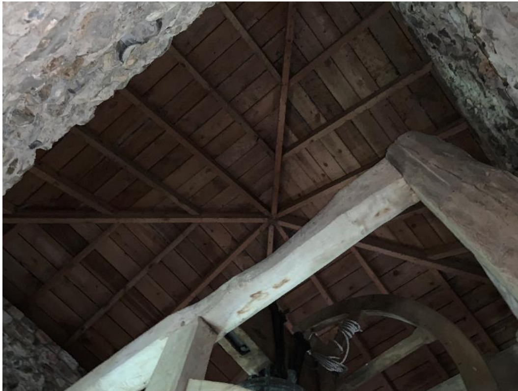
Photo 11. Tower roof interior.
