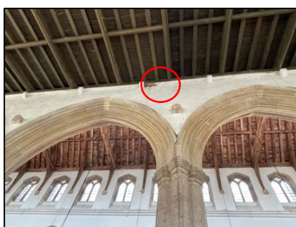
Figure 3 – Roost location in the south aisle Roost R2 in July 2021
