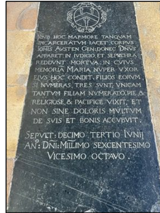
Figure 20 - Urine damage on the ledger stones, some fresh but lots of historical damage
