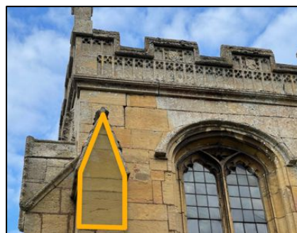
Figure 31 – Multi-chambered Kent type maternity box mounted on the buttress of the porch
