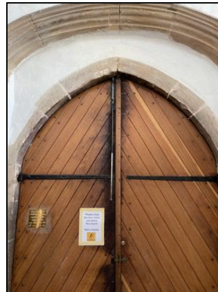
Figure 10 – Secondary access A3 via the southern porch door
