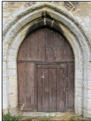
Figure 9 – Secondary access A2 via the western tower door
