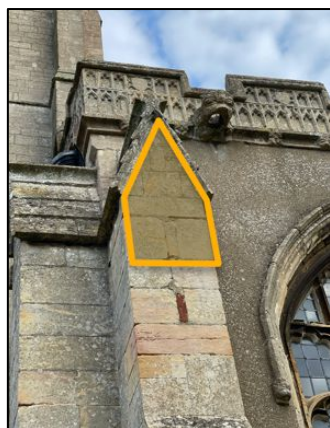
Figure 30 – Multi-chambered Kent type maternity box mounted to the south of the tower on the south-east corner of the south aisle buttress
