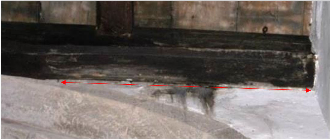
Photograph 2.1.5: A photograph of the droppings on the windowsill behind the reredos in 2013.
